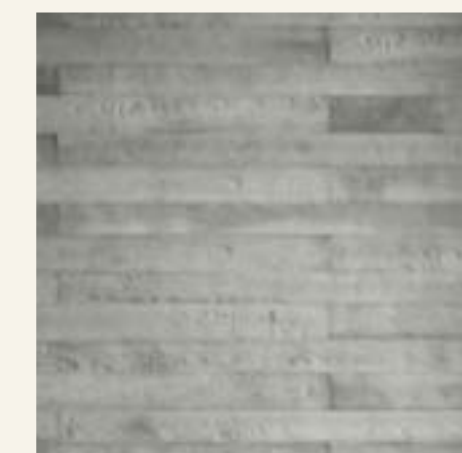
3. Wall Concrete decking Building Front
